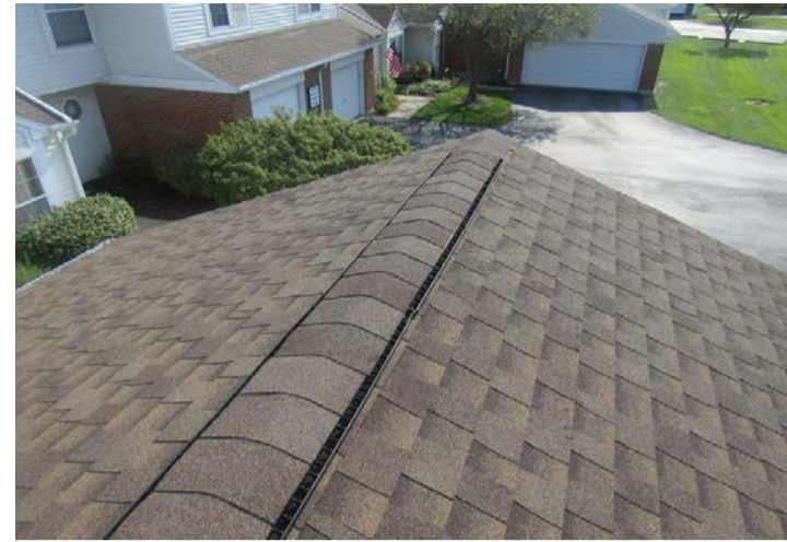
roof with asphalt shingles
