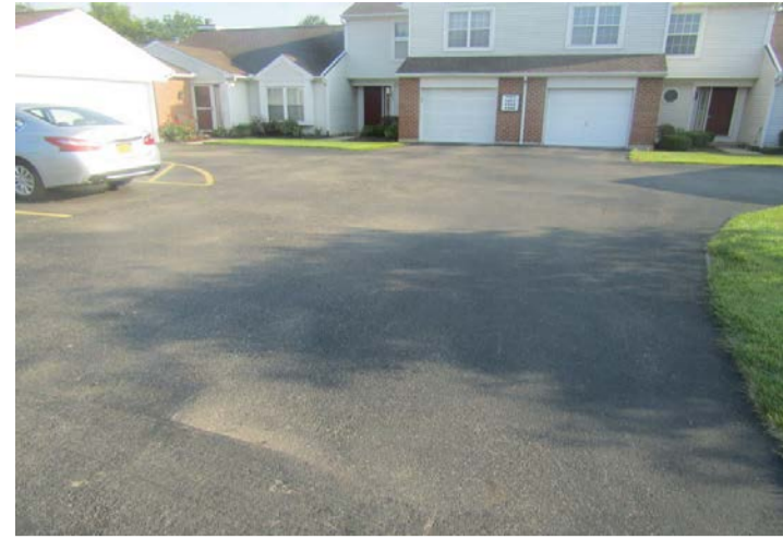
asphalt pavement at driveways
