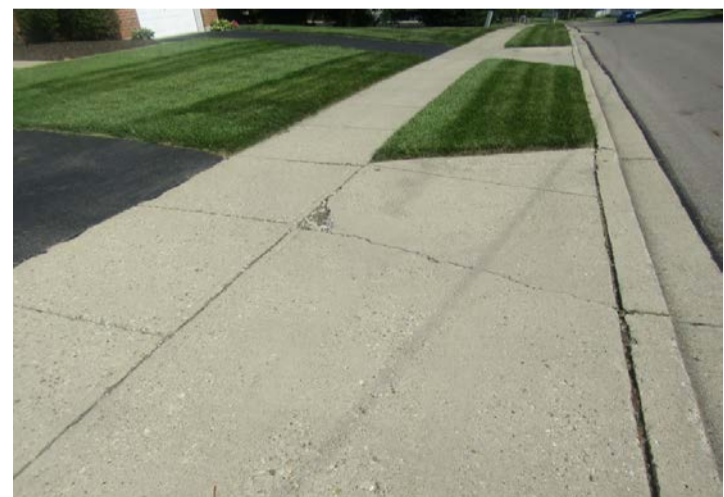
cracked concrete
