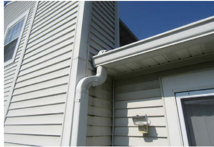
aluminum gutters and downspouts - rear
