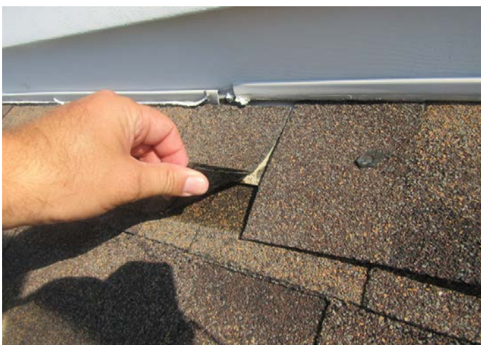
underlying shingles appropriately installed beneath flashing at roof to wall intersection
