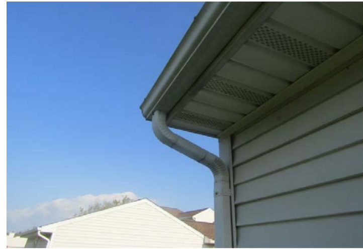
aluminum gutters and downspouts - front
