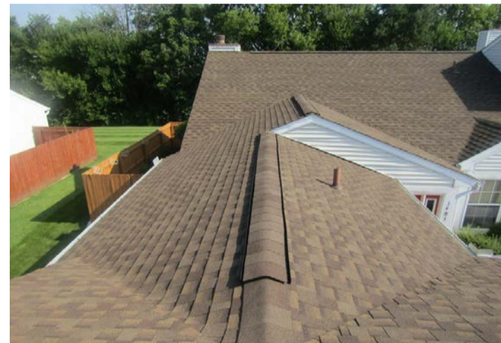
asphalt shingles and ridge vents with wind baffles
