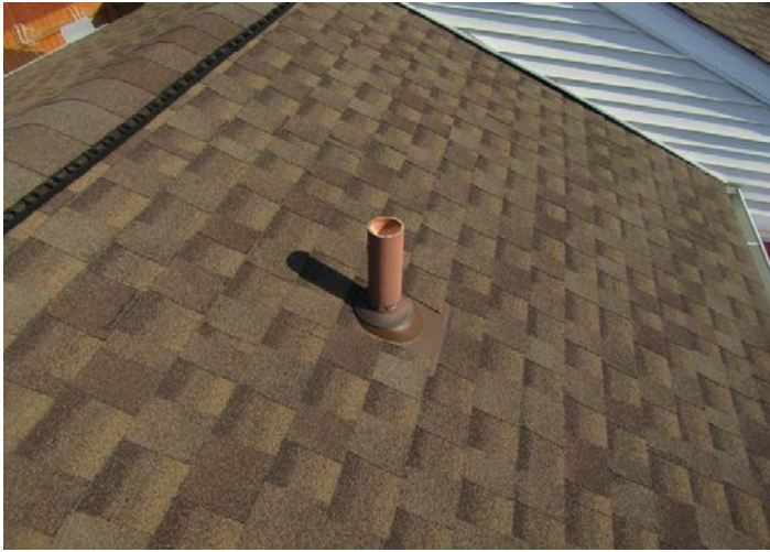
rubber and metal flashing at vent pipes
