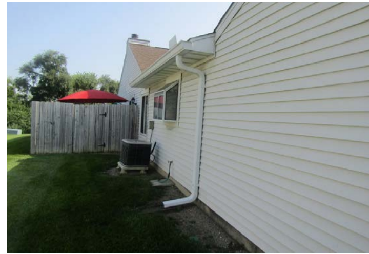
vinyl siding with clapboard double 4-inch profile
