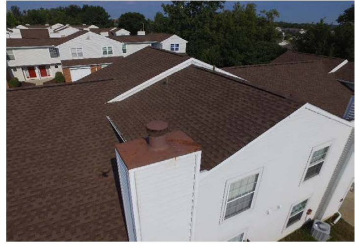
metal chimney chase cover
