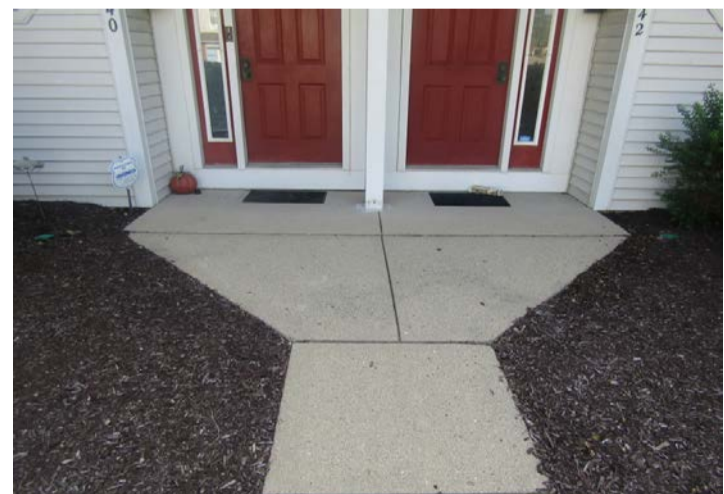
concrete sidewalk and stoops
