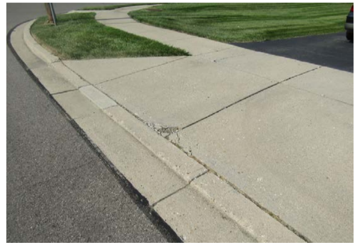
concrete disintegration
