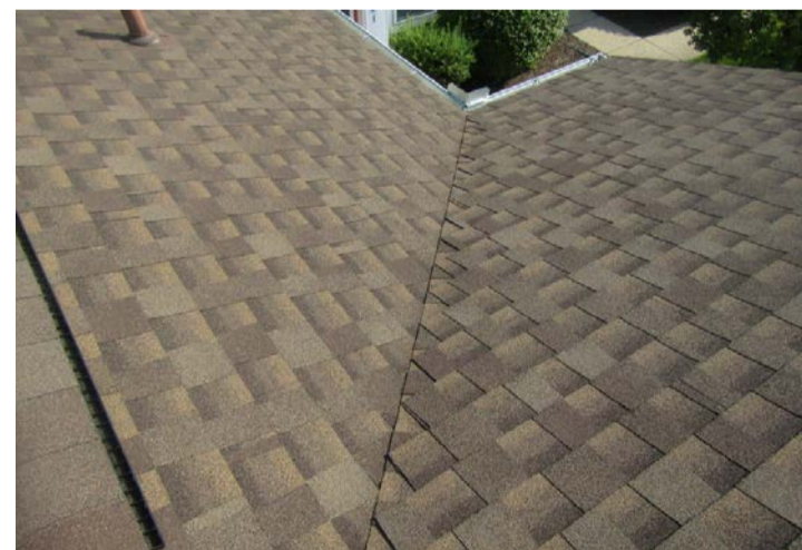
California style enclosed valleys
