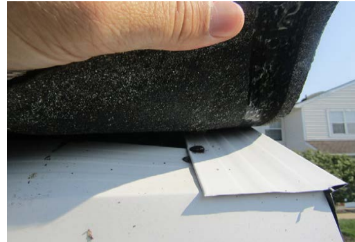
self adhering underlayment at gutter edge
